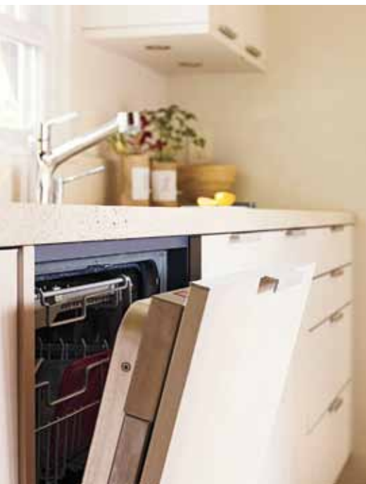
TOP LEFT: The Miele dishwasher is faced with a white panel to blend in with the rest of the cabinets.
